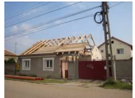
New roof at House of Joy
